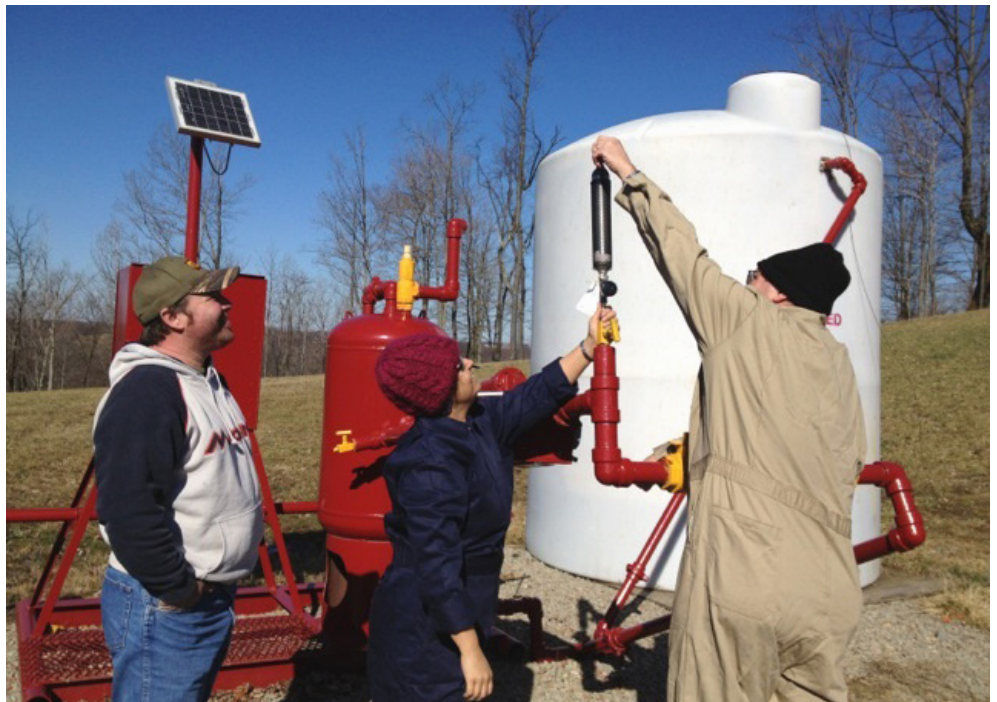
NETL’s Karl Schroeder, far right, collects natural gas samples to test for the presence of tracers detecting upward migration of gas from the hydraulically fractured Marcellus Shale. No tracers were detected in the process. Assisting were Shikha Sharma, a researcher with West Virginia University, and an unidentified well tender.
